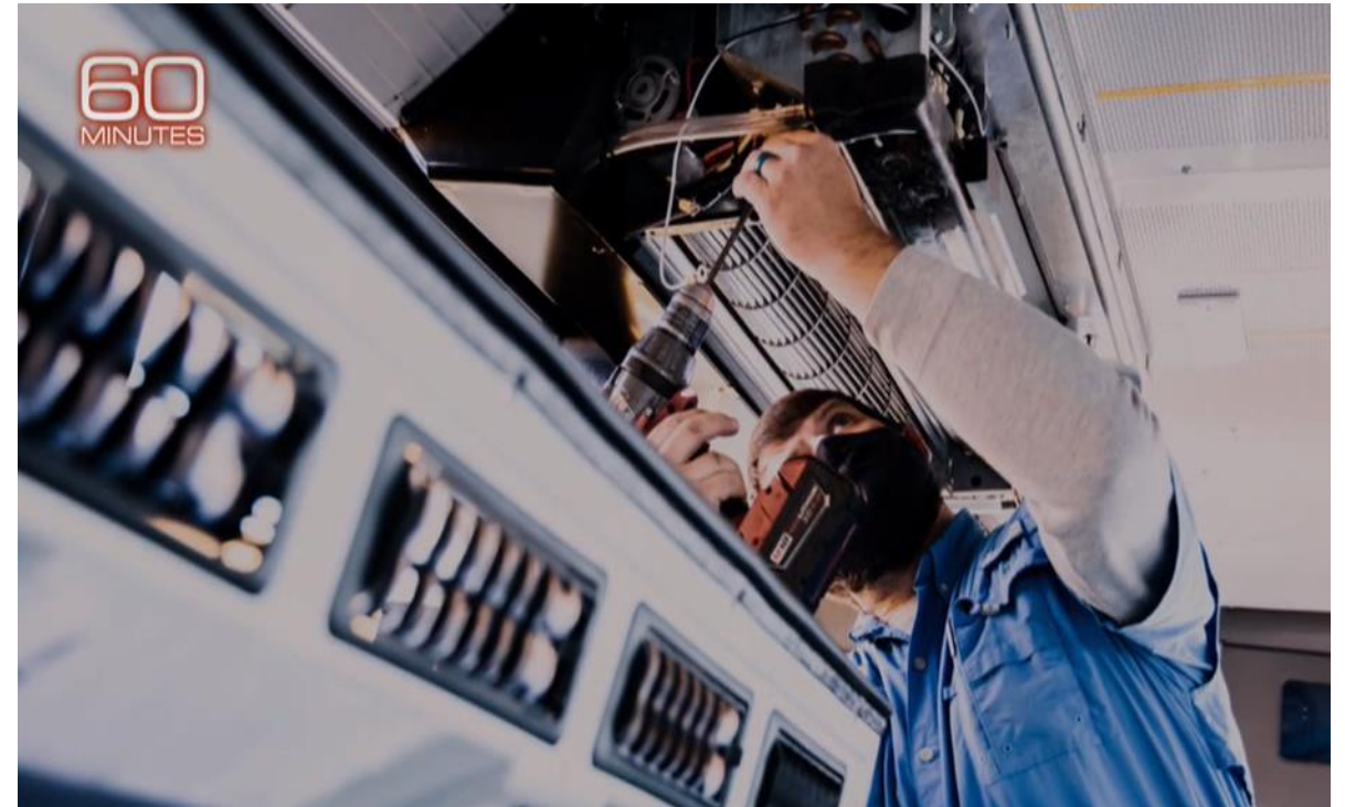
Custom Mobility Technician Installing NPBI Unit
